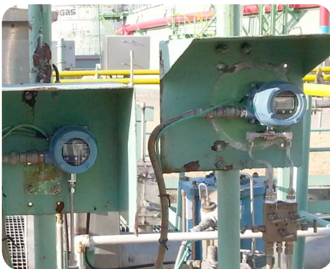
Control de gas natural
